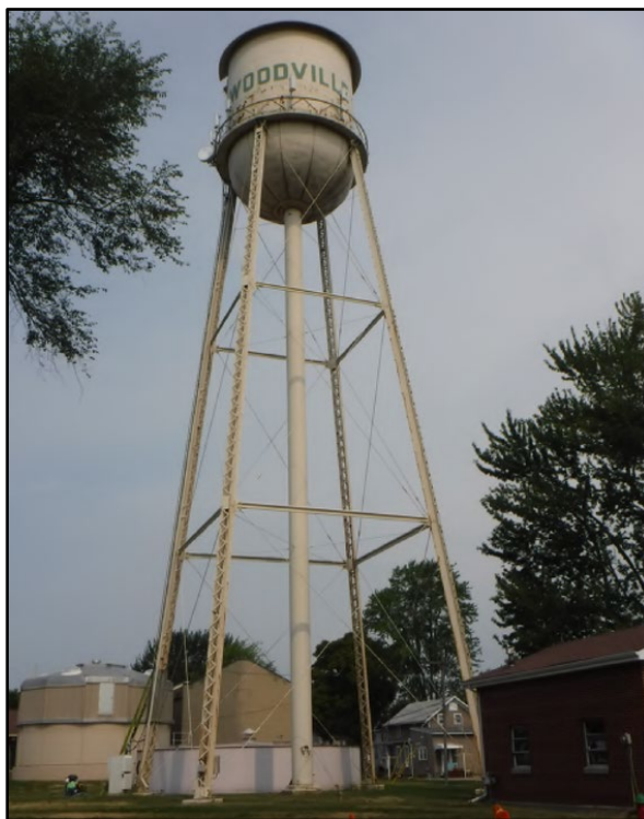
Figure 2. Woodville elevated water storage tank
